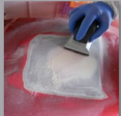
6 Block sand with either a P120 or a P180.
