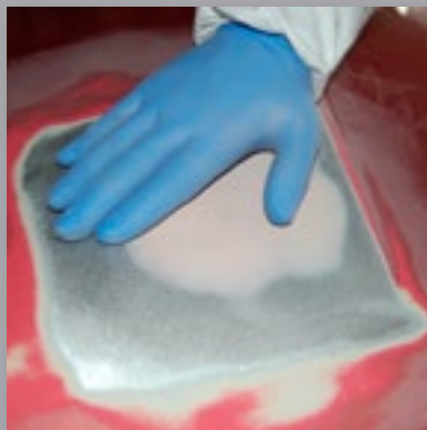
8 Final inspection ready for primer application process.
